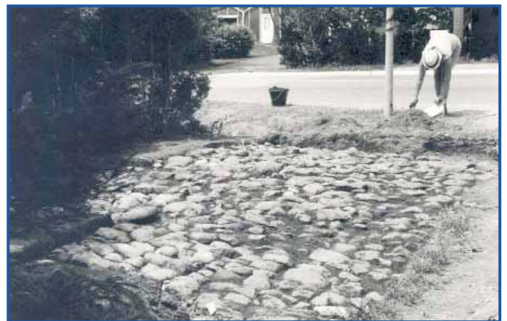
Blacksmith floor - Myrtle, Ontario
